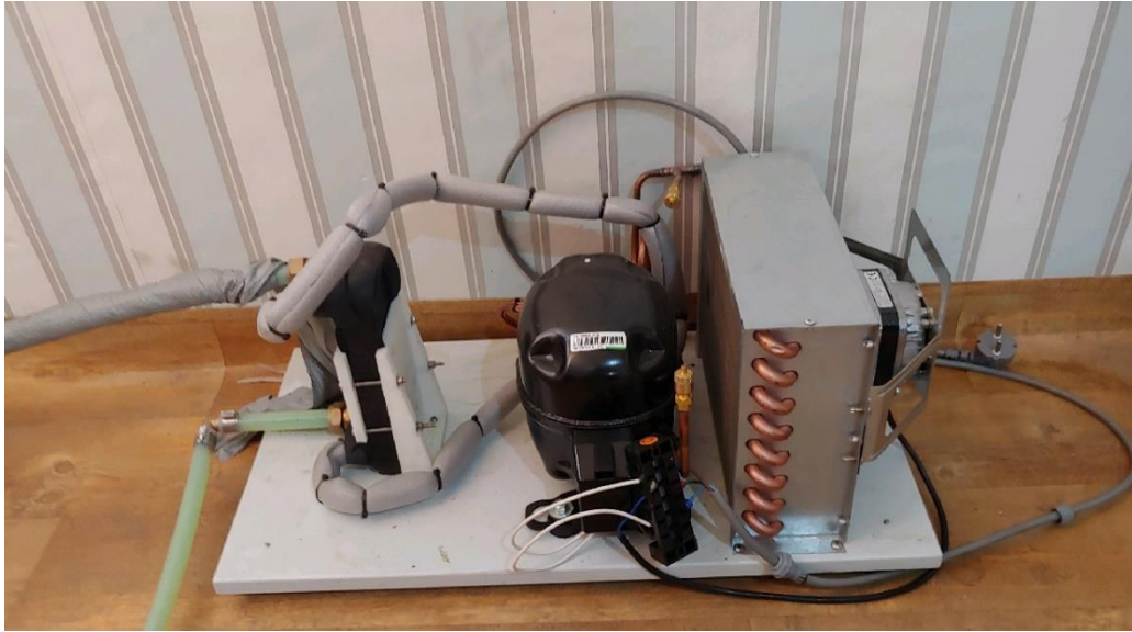
Figure 3. Chiller for cold water supply to the cold-water panels of the small cabins for one person
