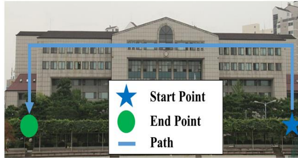
Figure 8. Front View of Hawdo Building and the Path of Experiment
