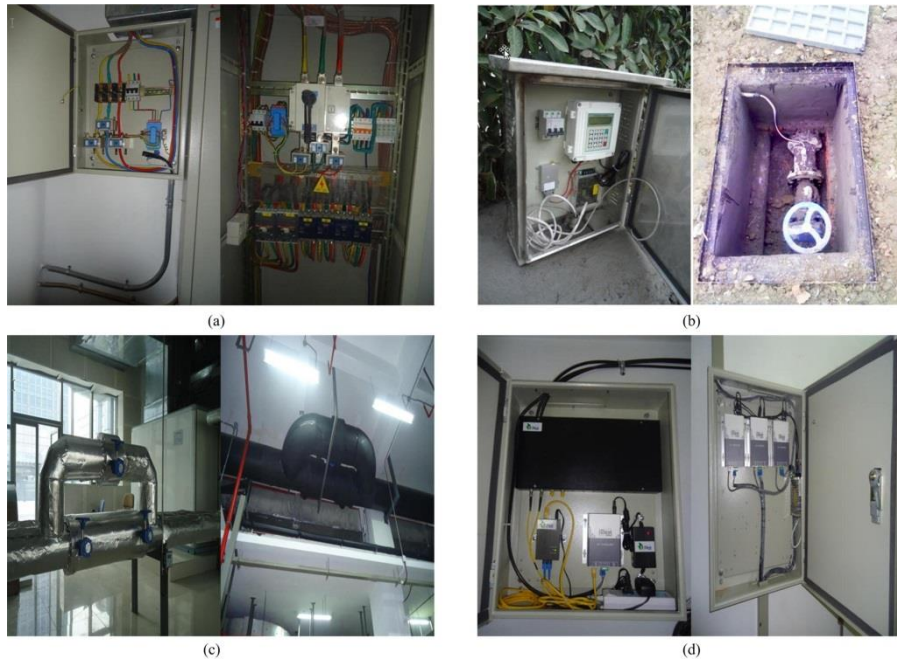
Figure 3: Installation of Measurement Meters and Data Collectors
