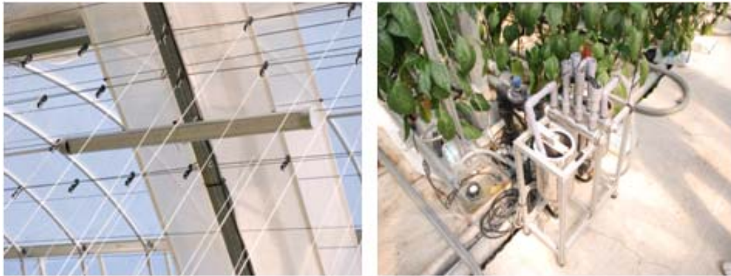
Figure 7. LED Lamp, Sun Shield and Warm water supply
