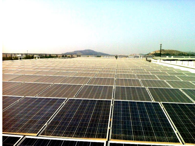
Figure 6. Laying of Solar Equipment
