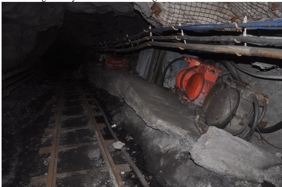
Figure 3.The Floor Heavein the Downhill Tunnel
