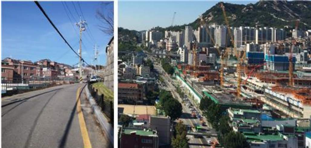
Figure 4. Situation of the Haengchon Area, 2015 Left: Haengchon-dong looking along the castle wall Right: Construction site of Donuimun New Town (Source: Photograph by author, L: January 2016, R: September 2015)
