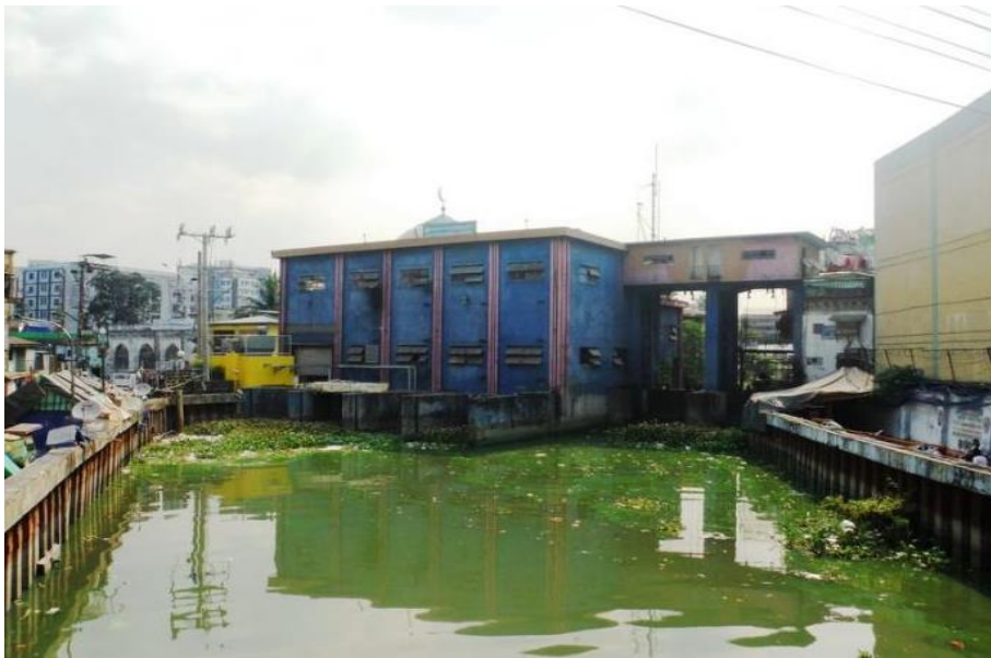
Figure 1. Existing Pumping Station in Manila
