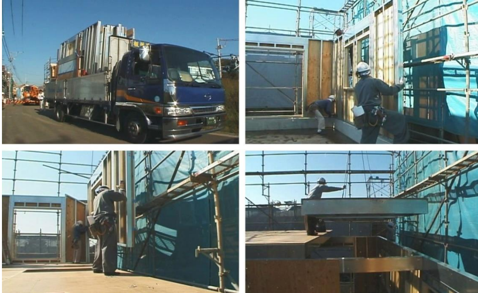
Figure 1. Construction Process of the Urban Residential Building Assembly in the Cold Regions in Sendai
