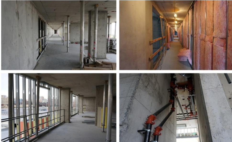
Figure 2. Internal and External Wall Technology of No Beam Floor and Light Steel Keel Structure Widely Used in Ottawa Apartment Residential
