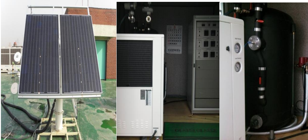
Figure 4. (left) View of the Experimental Setup of the PVT Collector and the (Middle and Right) Measuring Equipment
