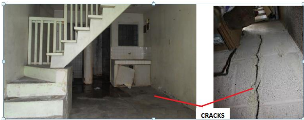
Figure 2. Cracks in Slabs
