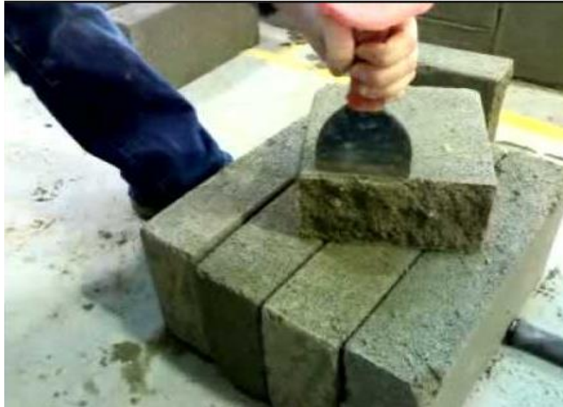
Figure 5. Half-High Split-Face Block at VMT Site
