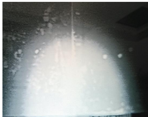
Figure 10. Thermal Imaging at 10 Sec After Heating
