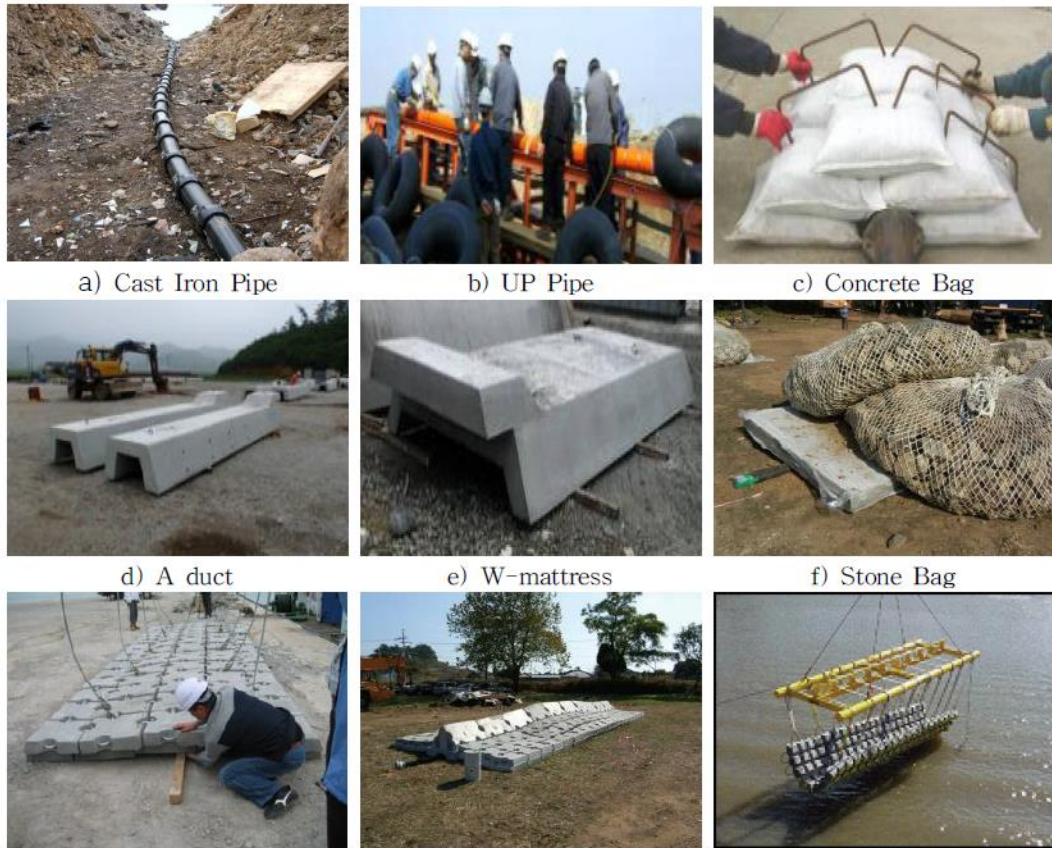
Figure 20. Protection Methods of Submarine Cable [9]
