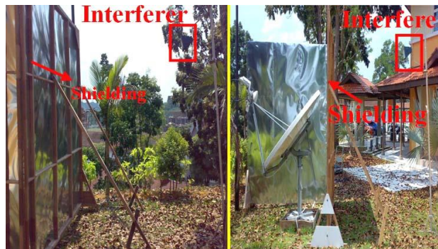
Figure 1. FSS Shielding using Zinc Sheet Material
