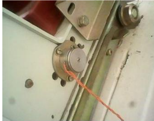
(b) Installation of angular displacement sensors
