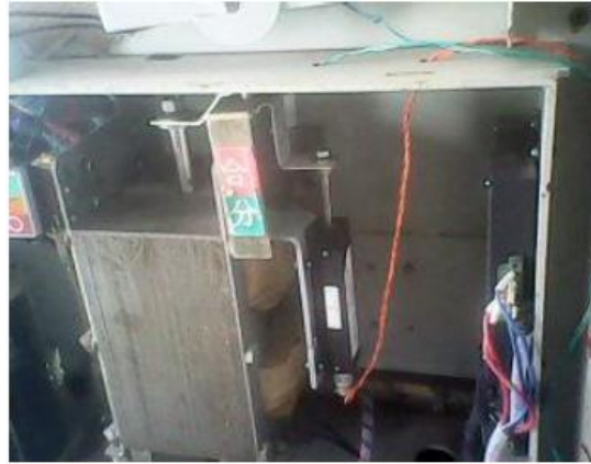
(a) Installation of linear displacement sensors
