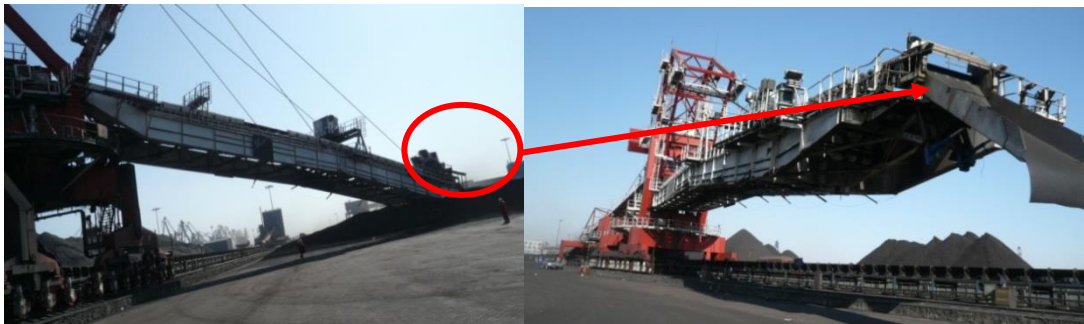
Figure 1. Change of the Stacker Reclaimer Structure (bucket wheel changed to be chute)
