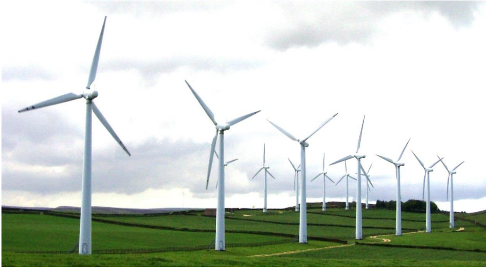
Figure 1. A Row of Turbines in a Wind Plant Located in Alberta, CA. This Wind Plant Contains 114 Horizontal Axis Wind Turbines (HAWTs), each Rated at 660 kW with a Rotor Diameter of 47m and Hub Height Approx 50m
