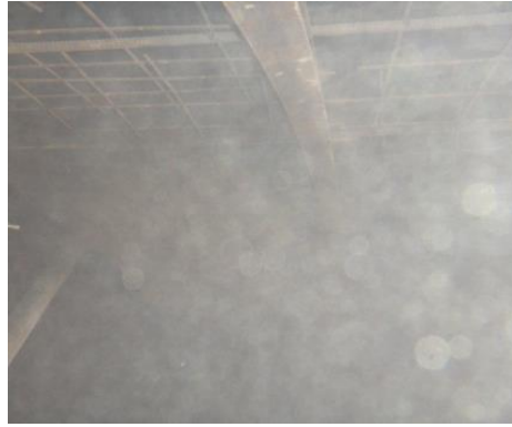
Figure 15. Field Dry Sprayed Concrete
