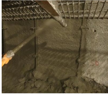
Figure 16. The Liquid Accelerator Matching Spraying Technology
