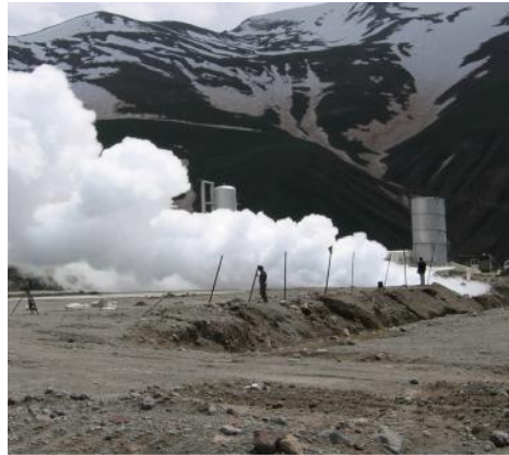
Figure 1. A View of the Power Plant under Construction in Meshkinshahr
